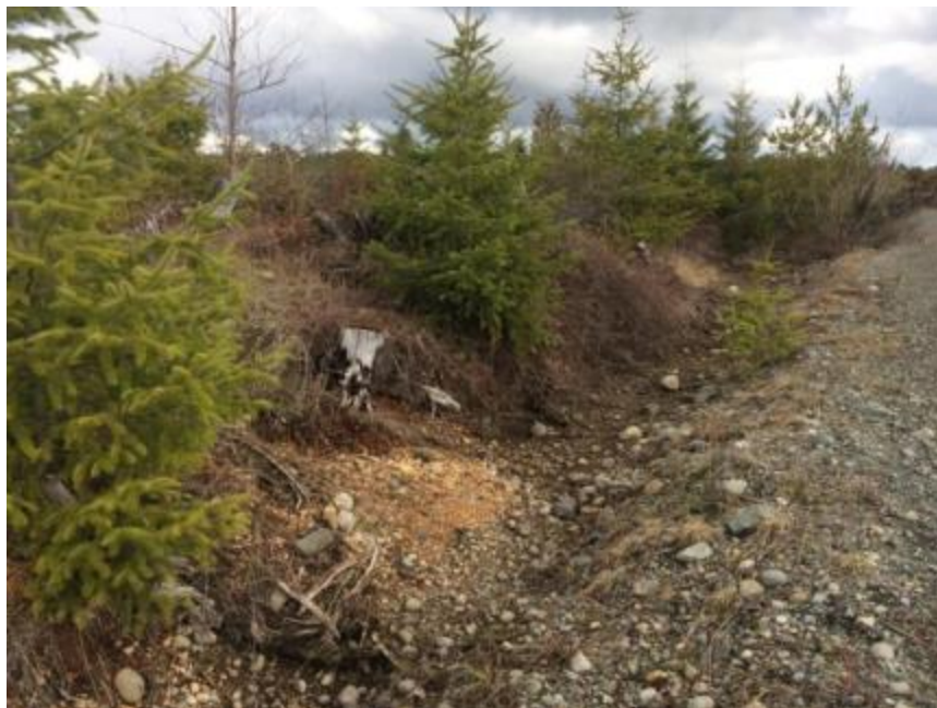
Photo 4. View of the roadside ditch portion of Watercourse 1 showing lack of flows in some sections.
