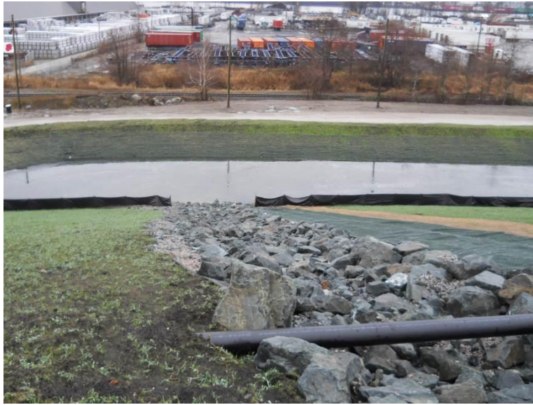
Photo 6-3: Delta Shake and Shingle Landfill Downchute
