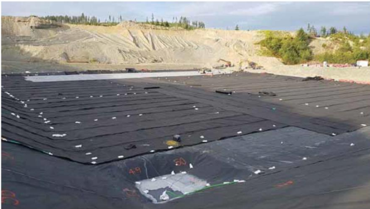
Photo 6-1: Leachate Sump Installation with Secondary HDPE Geomembrane and Leak Detection Geocomposite in Cell 1 East
