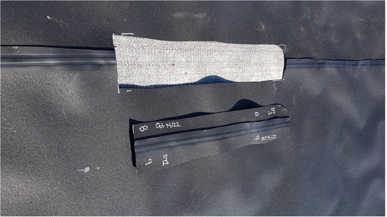
Photo 2 Typical Destructive Sample of Geomembrane Seam for Lab Testing
