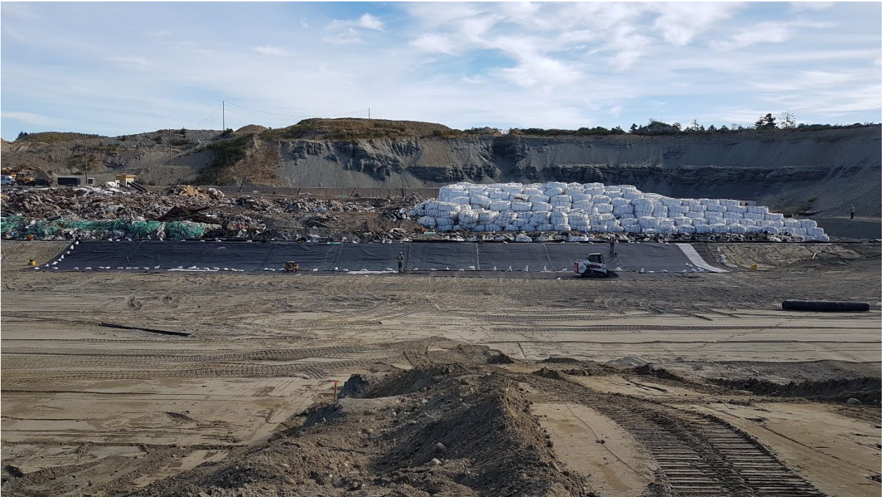
Photo 5 Primary Geomembrane Installation
