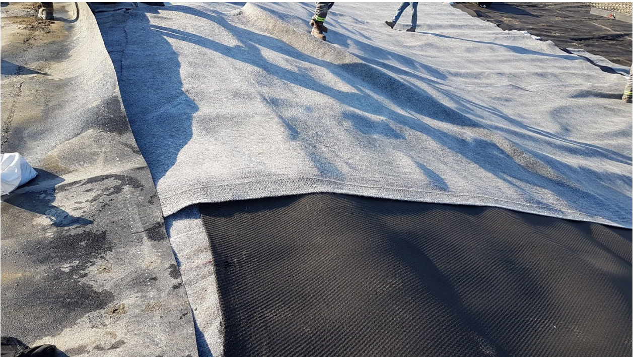
Photo 10 Installing GCL on top of Geocomposite
