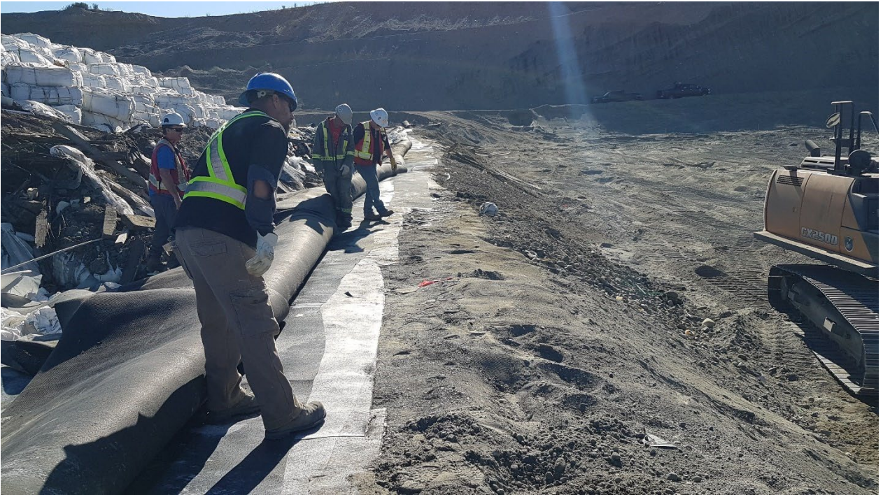
Photo 1 Installing Non-Woven Geotextile
