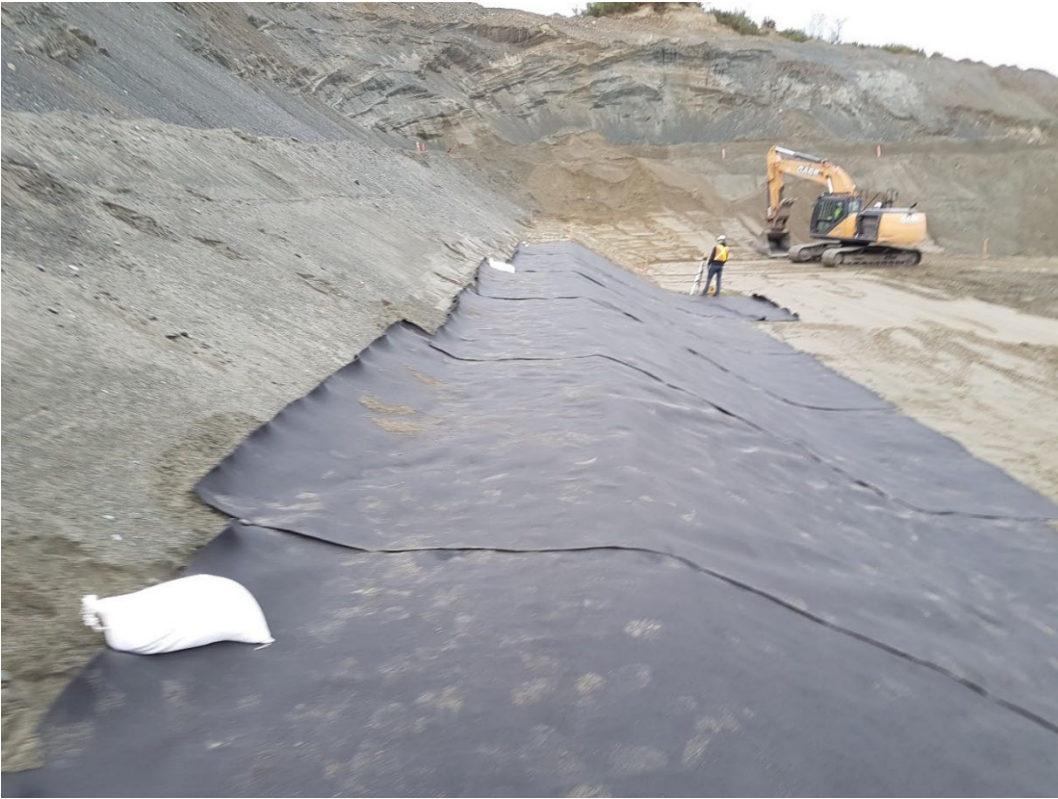
Photo 13 Deploying Non-Woven Geotextile
