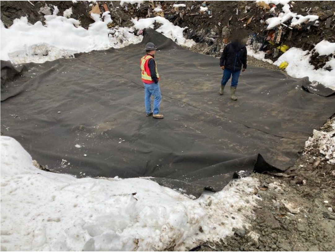
Photo 25 Completed repair to damaged liner area (November 18, 2022)
