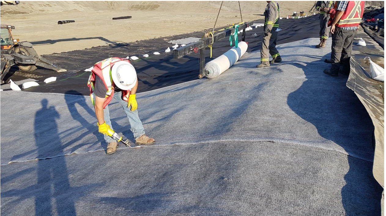
Photo 6 Seaming GCL and Primary Geomembrane Installation
