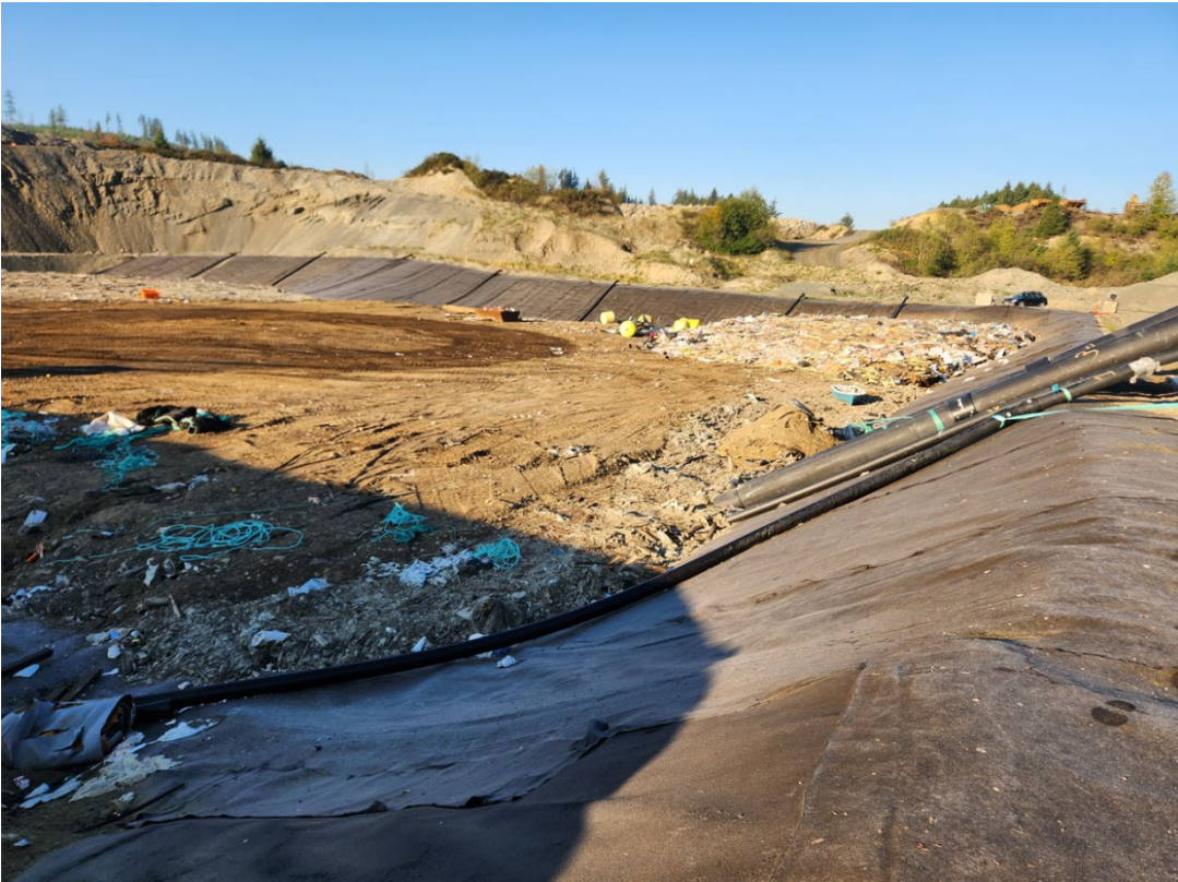
Photo 28 Cell 1 West from northeast corner (September 22, 2023)
