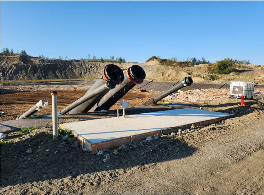
Photo 26 Leachate and leak detection risers / concrete poured for pump station (September 22, 2023)
