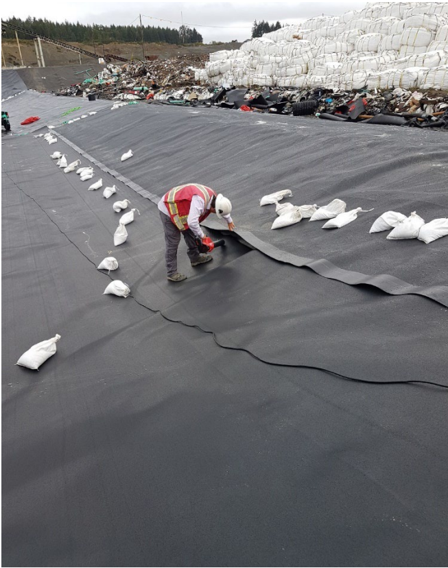
Photo 16 Seaming the Geomembrane
