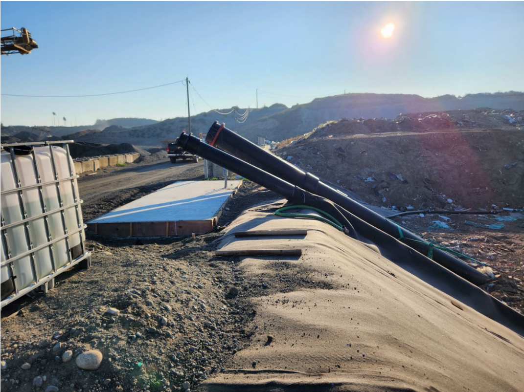
Photo 25 Leachate and leak detection risers / concrete poured for pump station (September 22, 2023)
