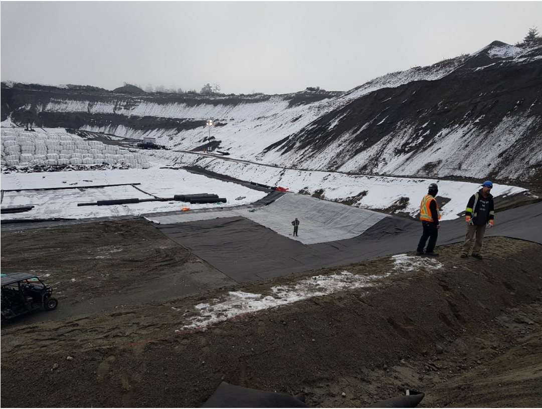
Photo 23 Deploying Primary GCL on top of Geotextile
