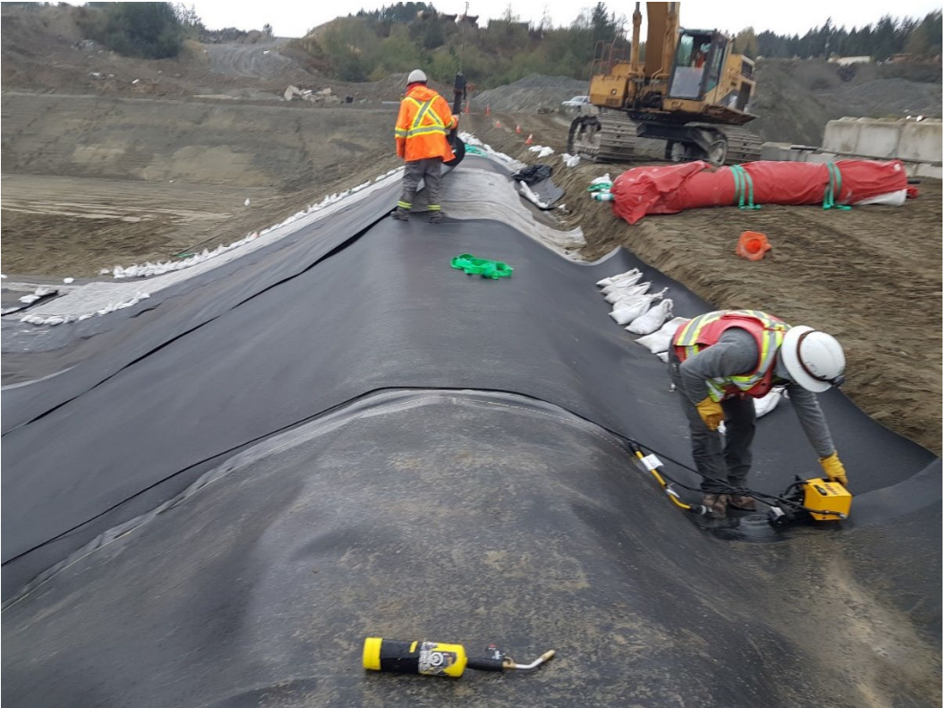
Photo 14 Geomembrane Welding in Liner Anchor Trench
