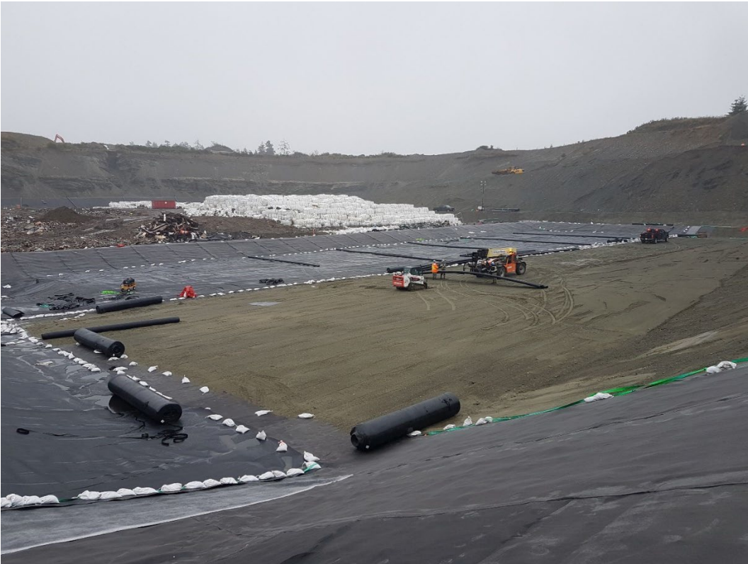
Photo 21 Placing Leachate Collection Pipes
