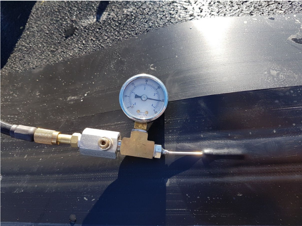
Photo 22 Geomembrane Seam Pressure Test
