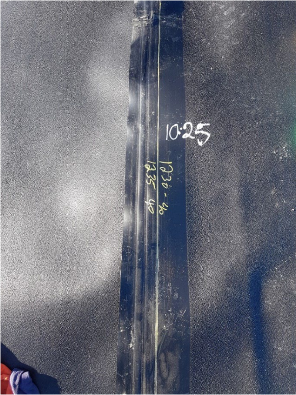
Photo 24 Geomembrane Seaming
