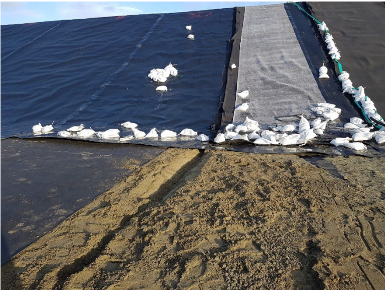
Photo 20 Deploying the secondary GCL on the North Berm
