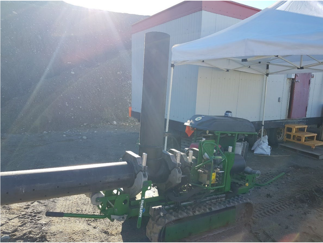
Photo 18 HDPE Pipe Fusion Machine
