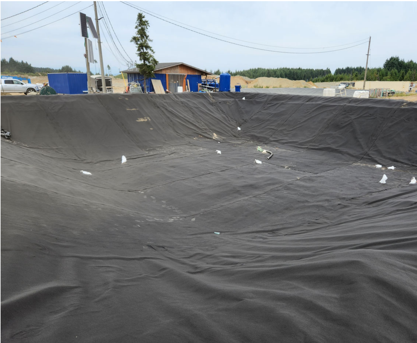
Geotextile on effluent pond before HDPE
