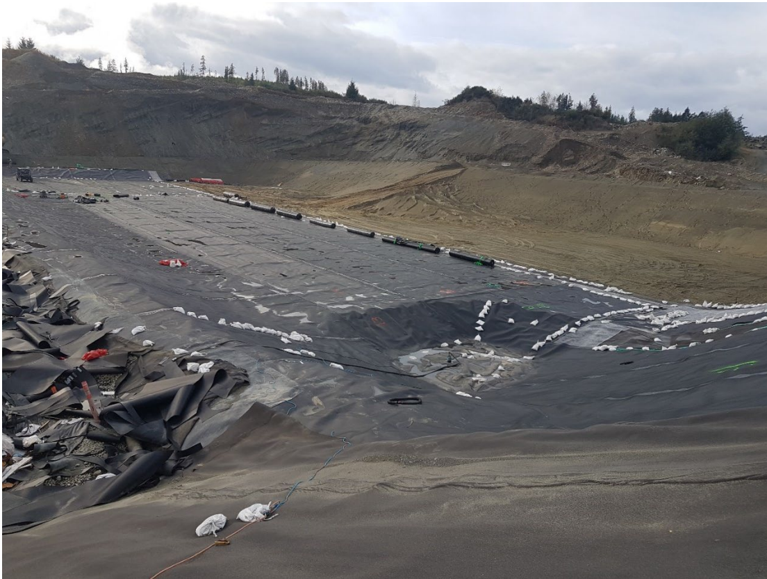
Photo 12 Leachate Sump with Primary Geomembrane
