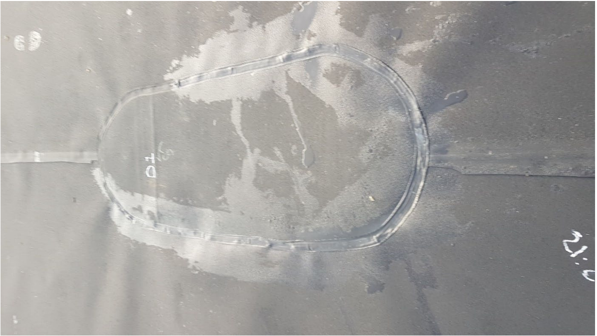
Photo 7 Typical Geomembrane Repair
