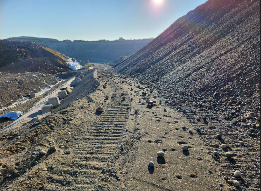
Photo 30 South end of Cell 2 (September 22, 2023)
