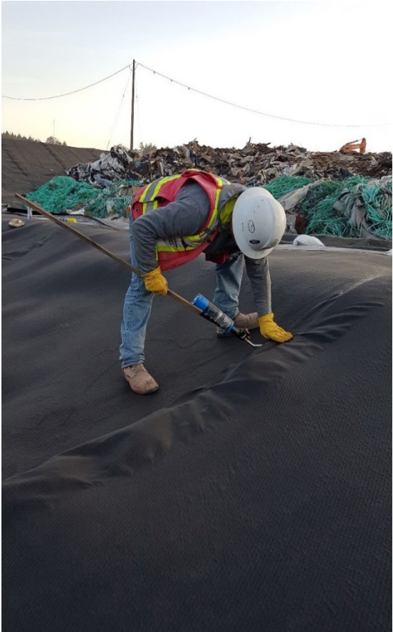
Photo 8 Seaming Geomembrane
