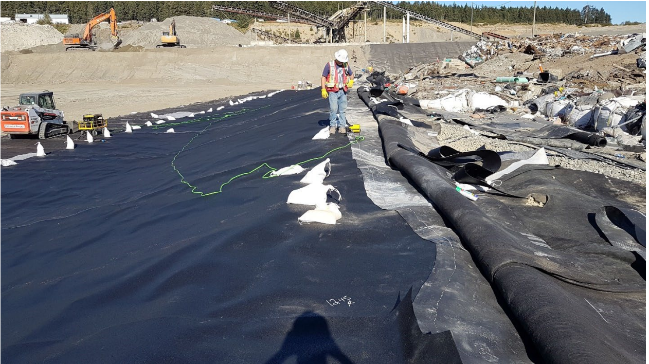
Photo 3 HDPE Liner Welding Cell 1 West to Cell 1 East Tie in
