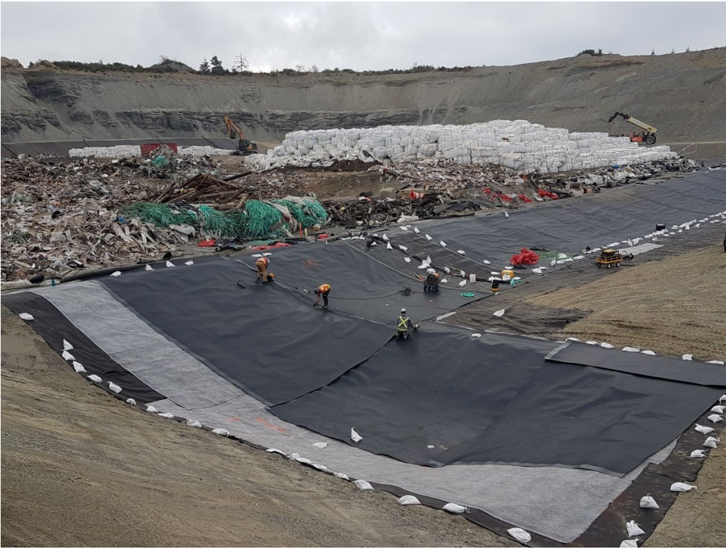
Photo 15 Seaming the Geomembrane
