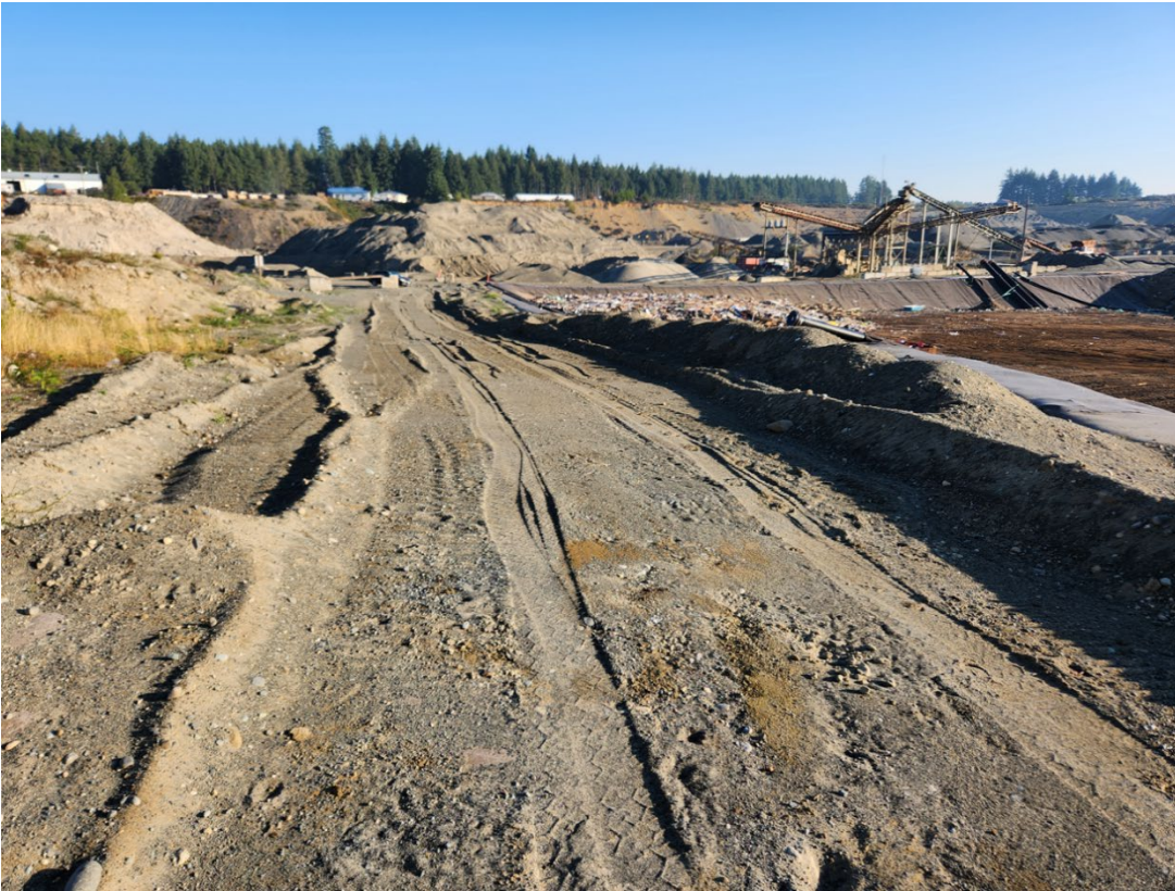
Photo 29 West perimeter road. Berm to prevent surface water run-on visible on right side of photo (September 22, 2023)
