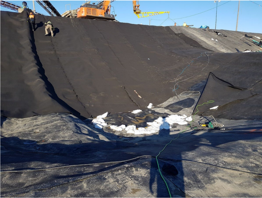
Photo 17 Seaming Geocomposite on the North Berm
