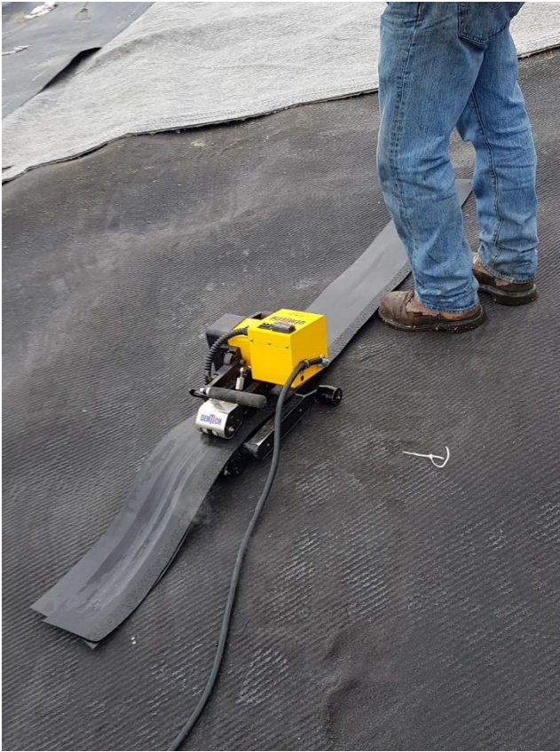
Phot 11 Test Weld
