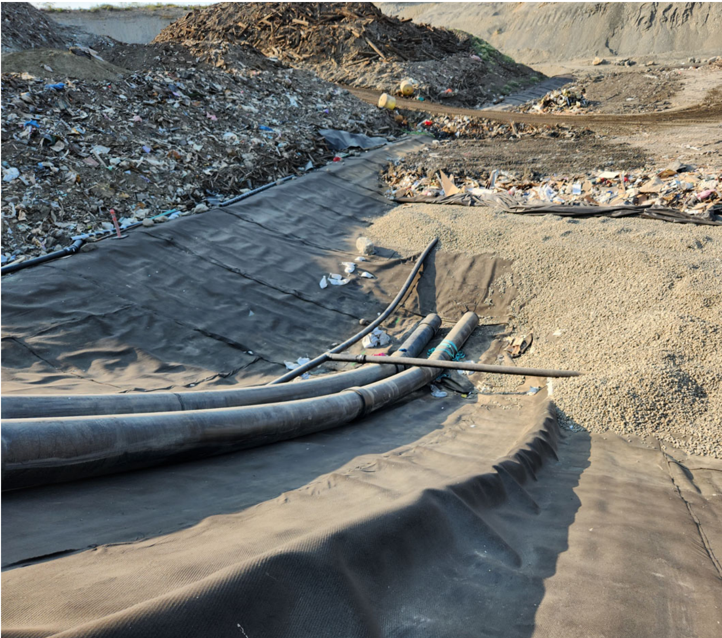
Cell 1 West Sump ready for drainrock installation
