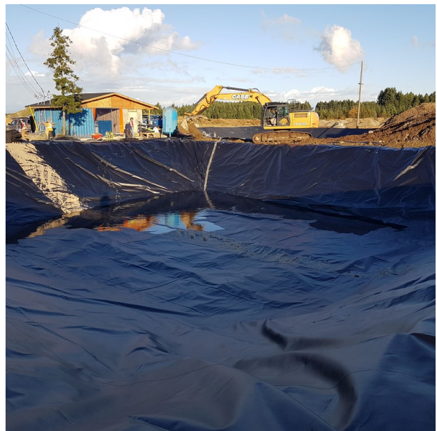
Photo 4 Effluent pond after reconstruction
