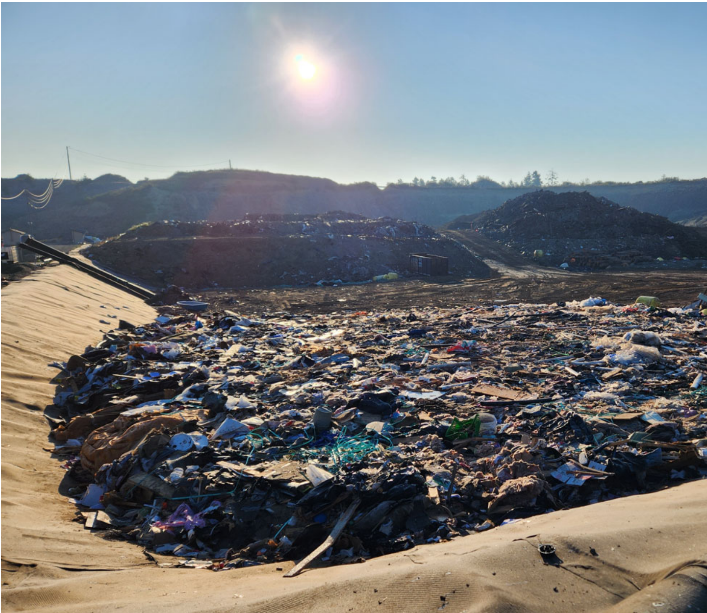
Cell 1 West viewed from northwest corner
