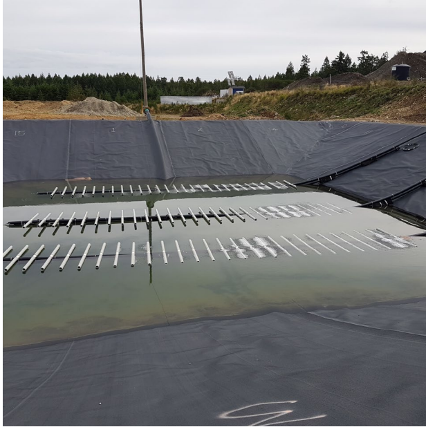
Photo 1 Aerated Treatment Pond
