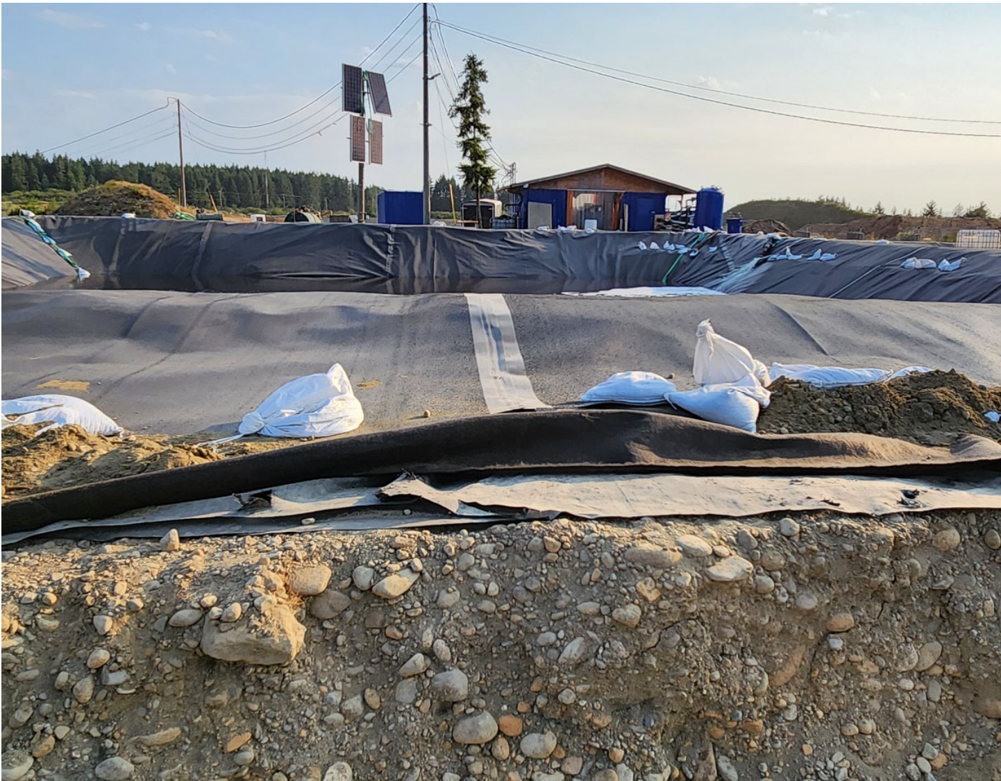
HDPE liner with previously installed liner visible
