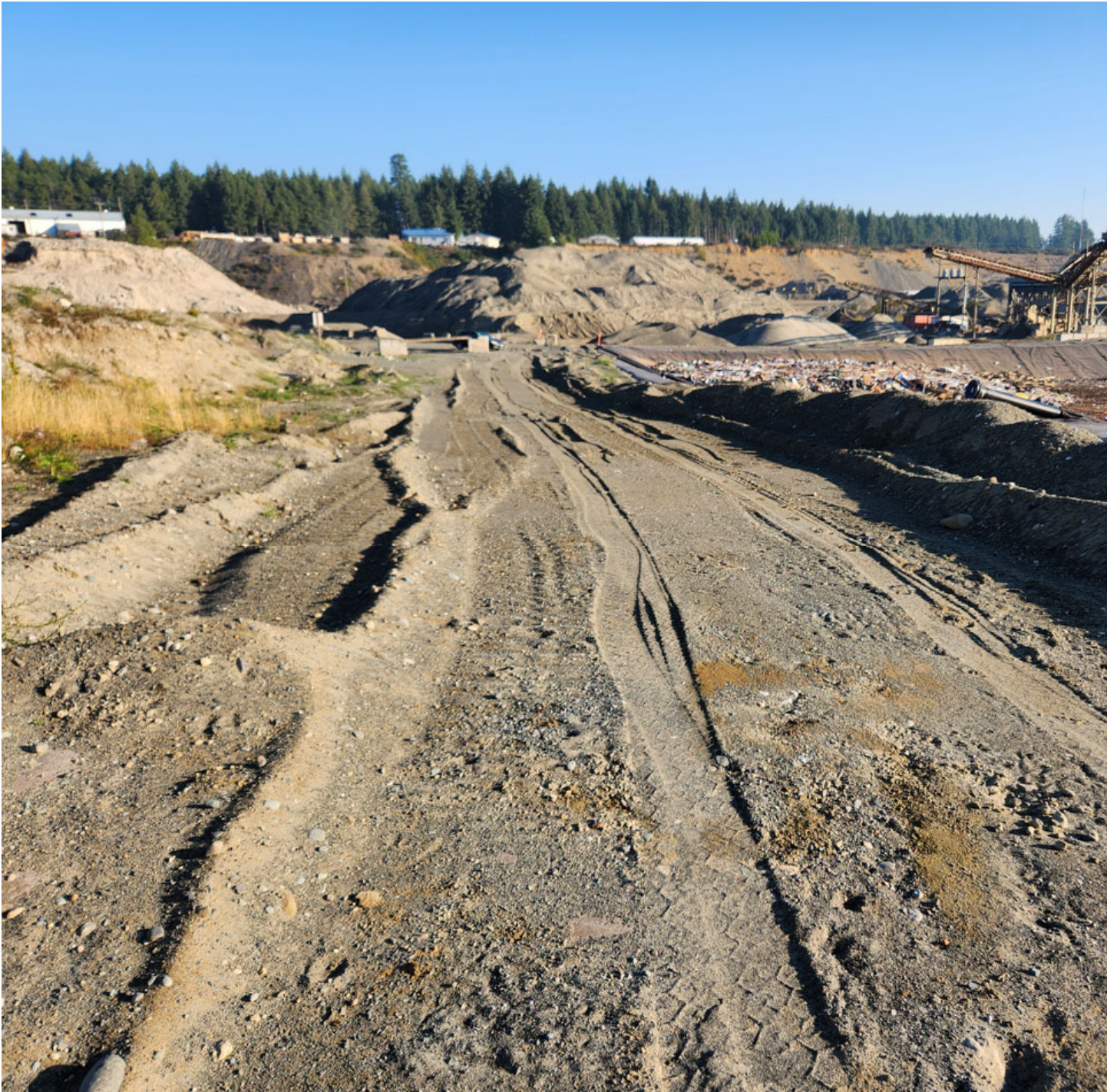
West perimeter road. Berm to prevent surface water run-on visible on right side of photo
