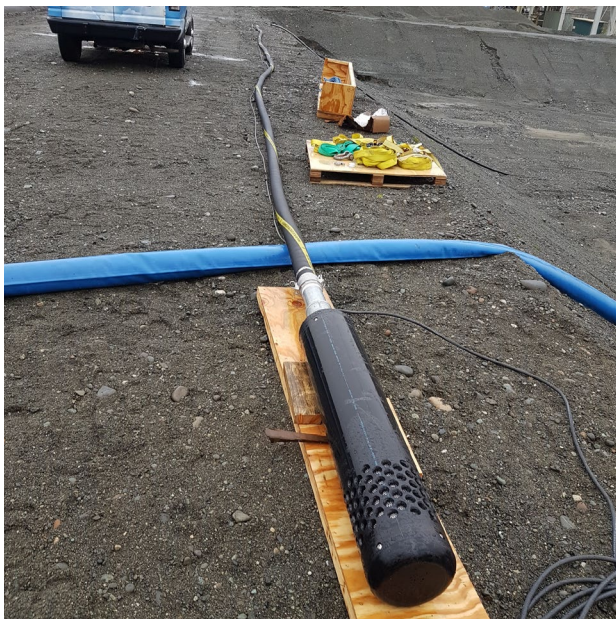
Photo 3 Submersible landfill leachate pump
