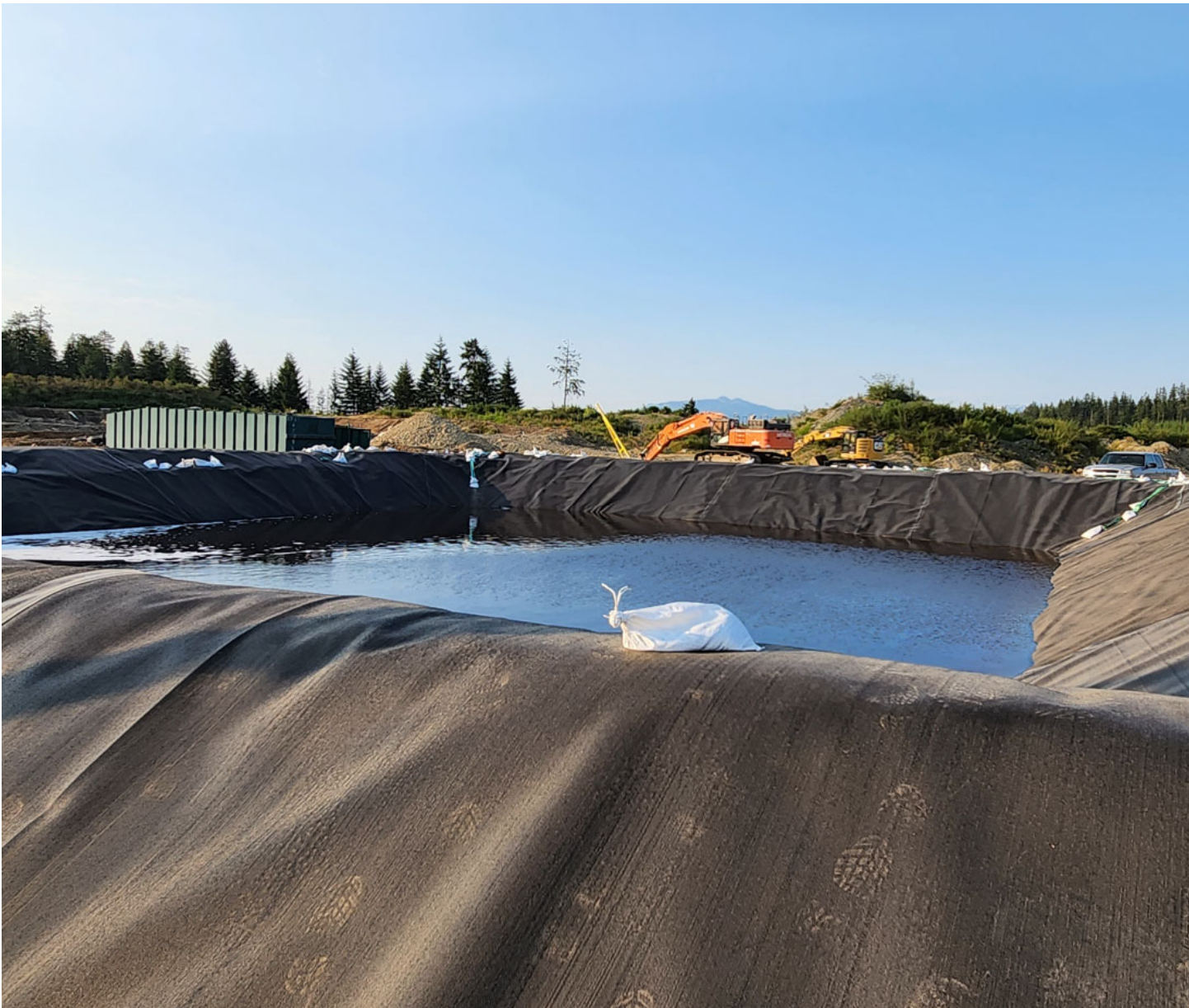
Effluent pond after HDPE installation
