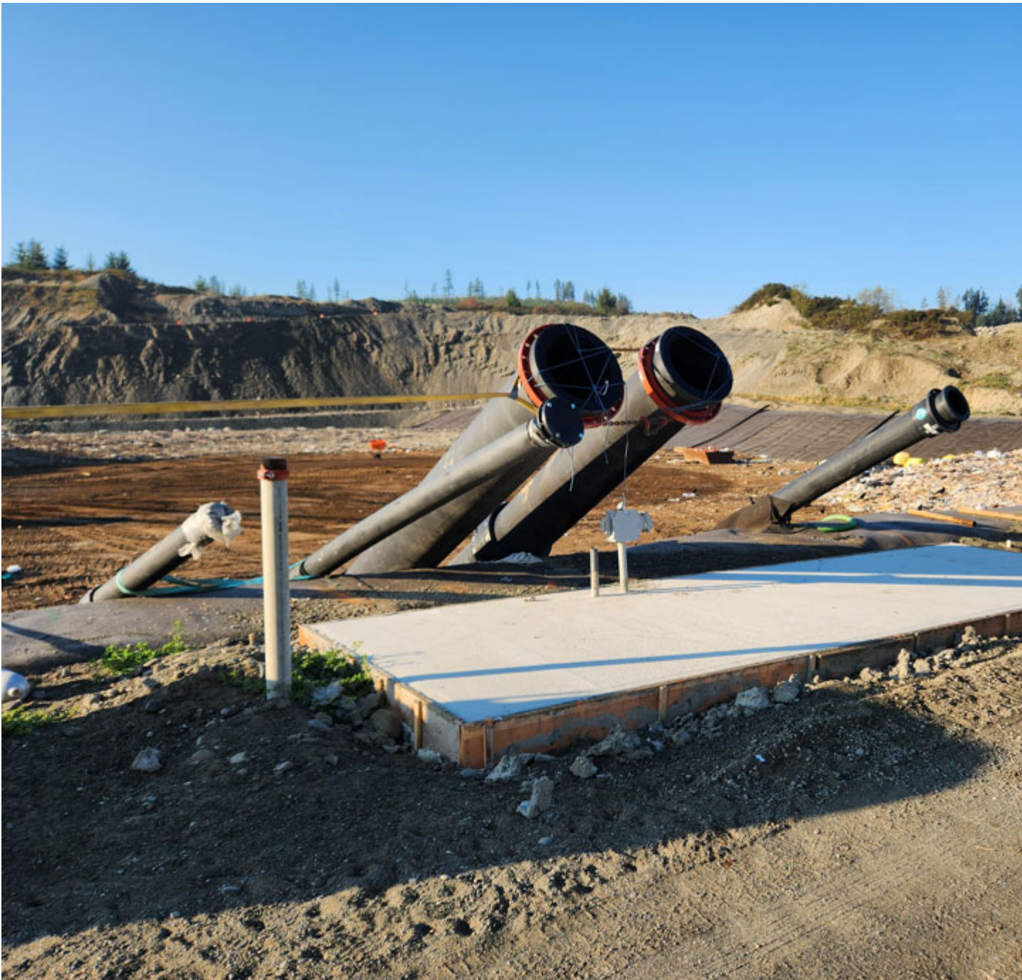
Leachate and leak detection risers / concrete poured for pump station
