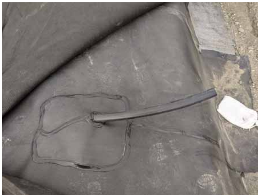
Photo 28 Typical Geomembrane Penetration Boot
