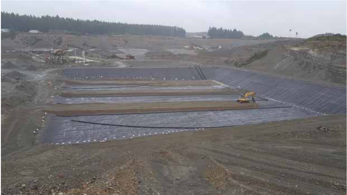
Photo 25 Completing Third 900 mm Drainage Layer Lift
