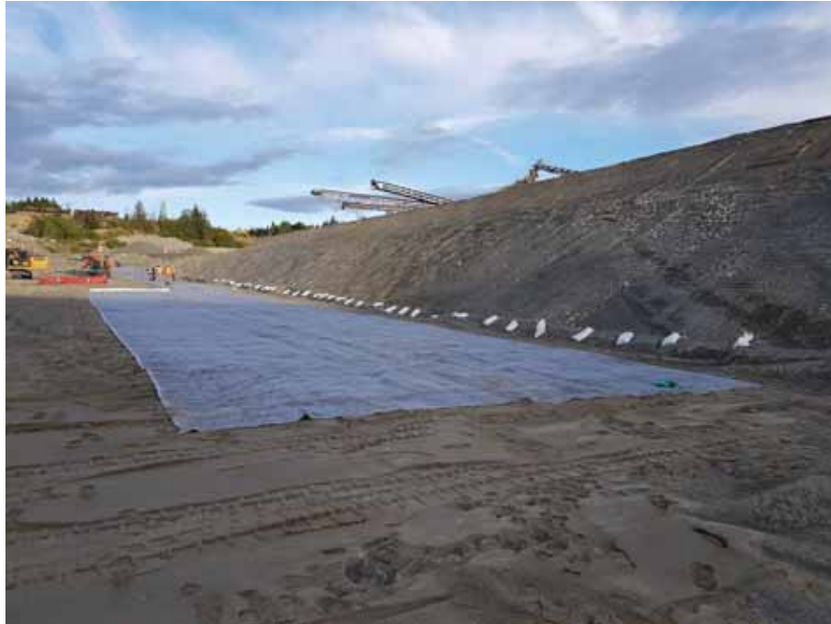
Photo 7 GCL Installation
