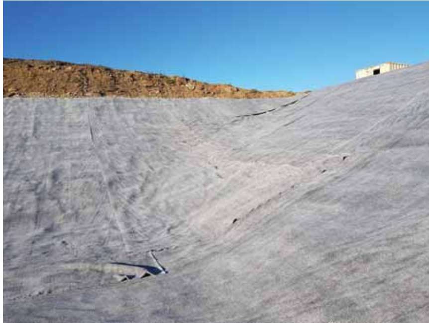
Photo 3 Leachate Treatment Pond GCL Installation
