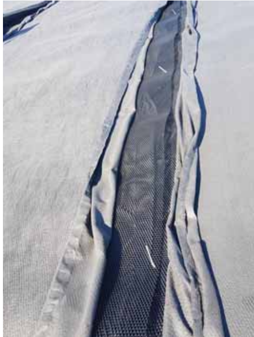
Photo 13 Typical Drainage Geocomposite Cable Ties
