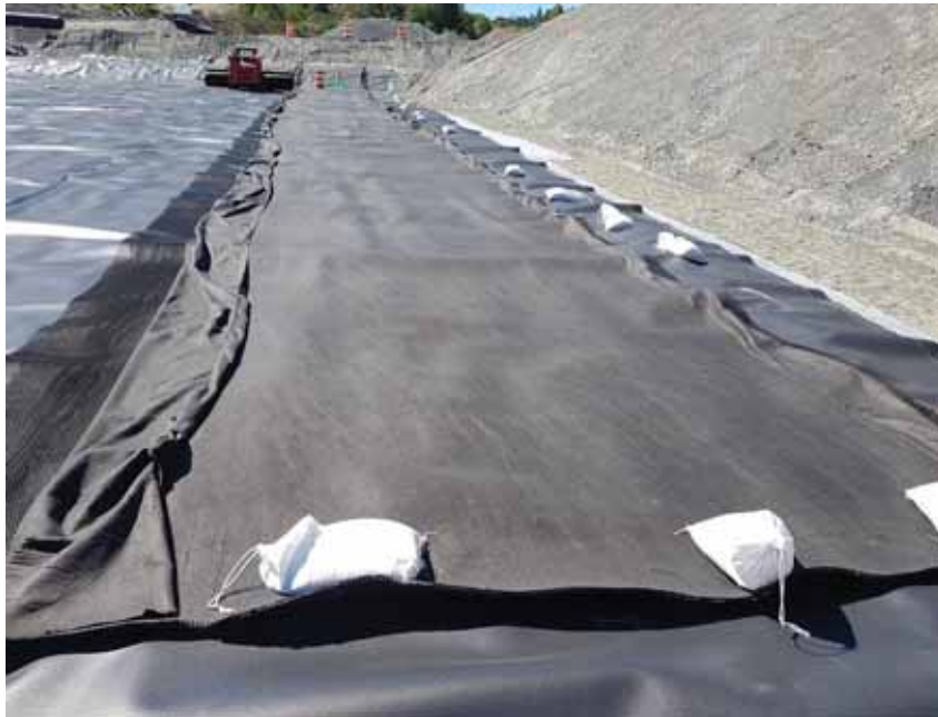
Photo 12 Drainage Geocomposite on top of Primary Geomembrane
