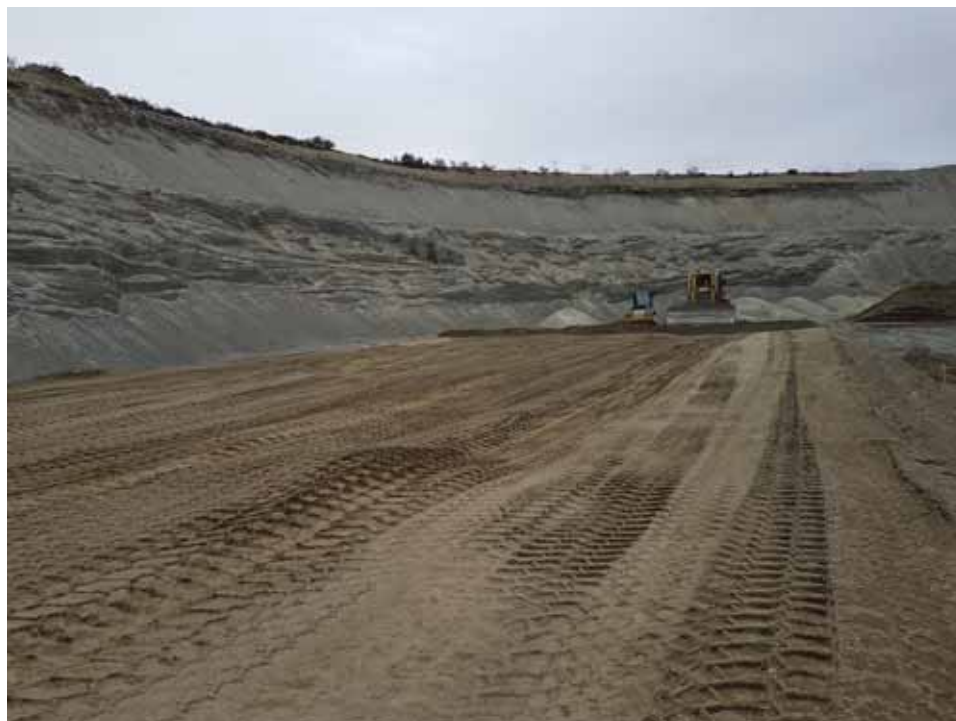
Photo 2 Constructing West Berm
