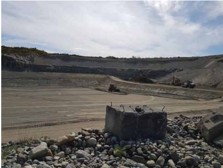
Photo 3 Placing Bedding Sand
