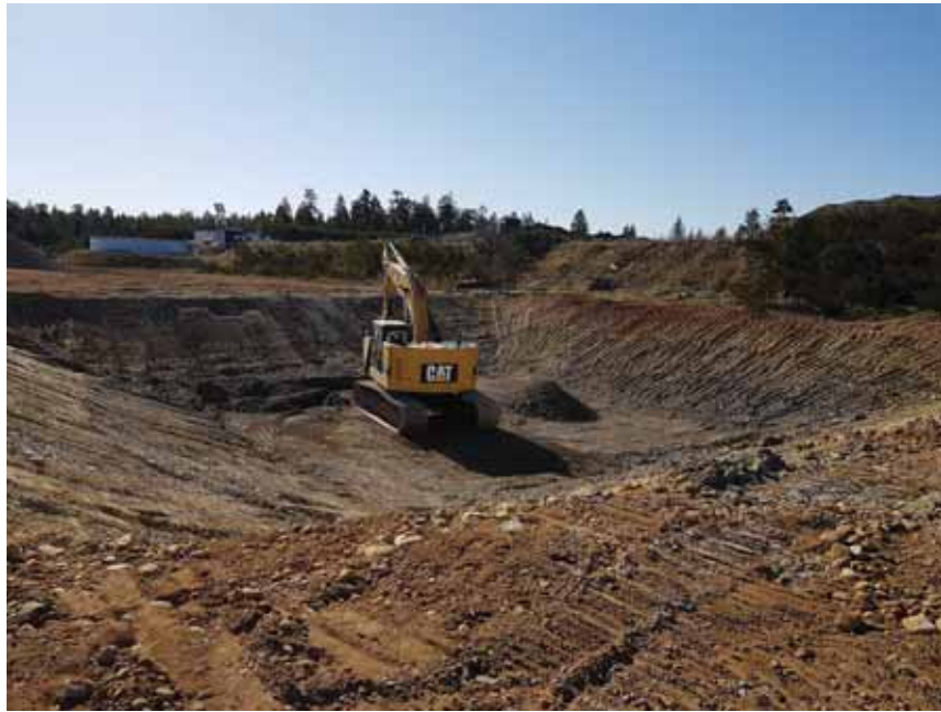
Photo 1 Leachate Treatment Pond Excavation
