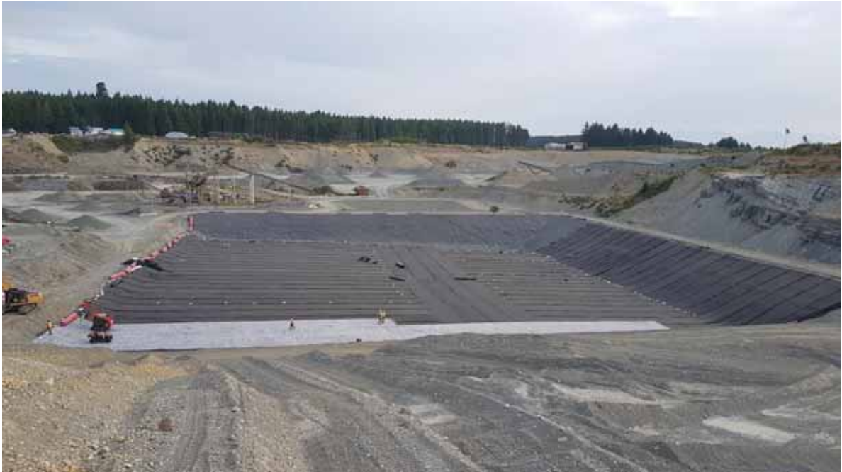
Photo 15 Installing GCL on top of Geocomposite
