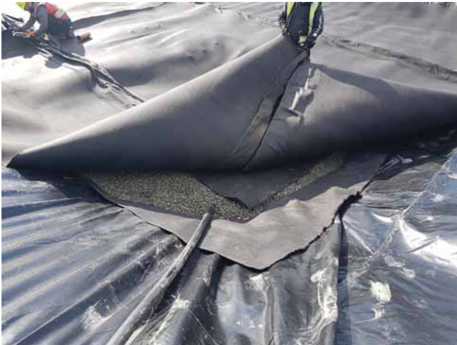
Photo 10 Treated Effluent Holding Pond Leak Detection
