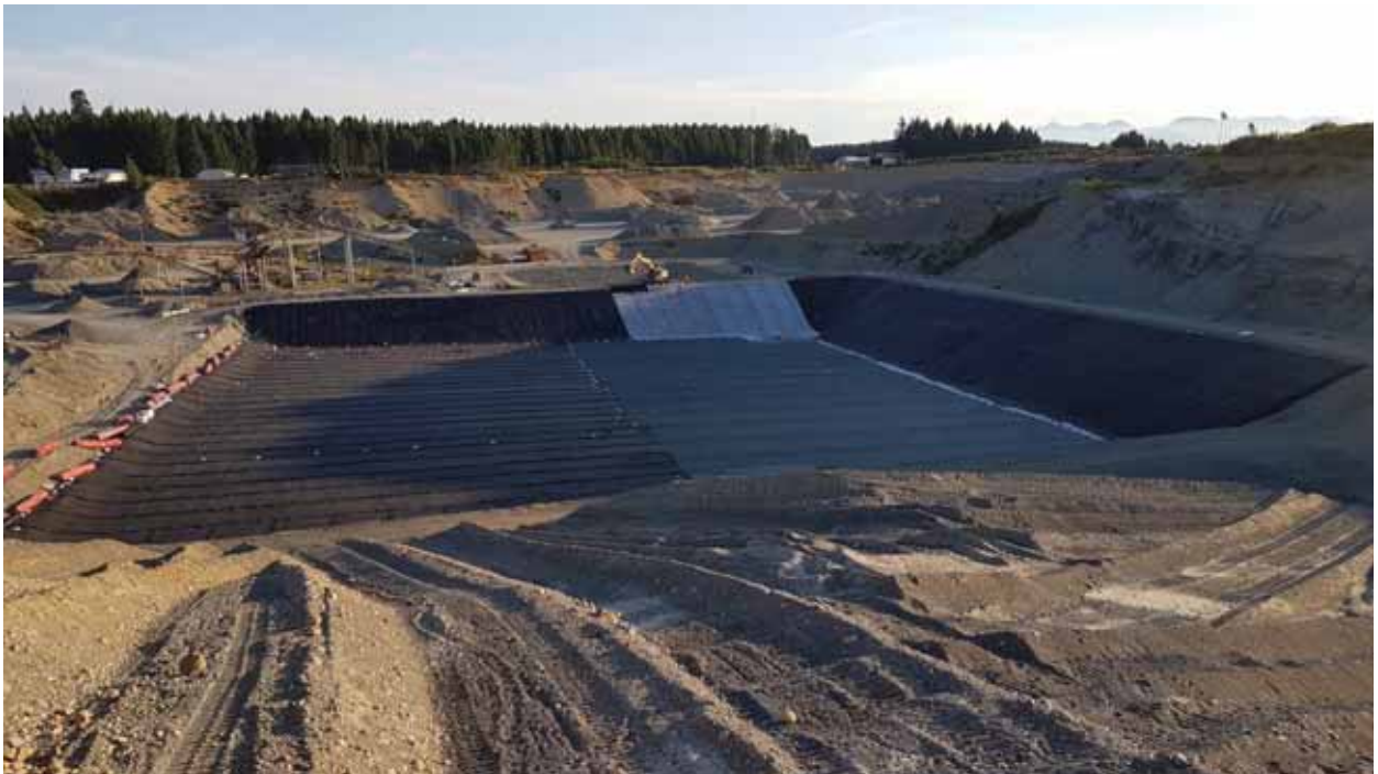
Photo 14 Installing Geomembrane on North Berm
