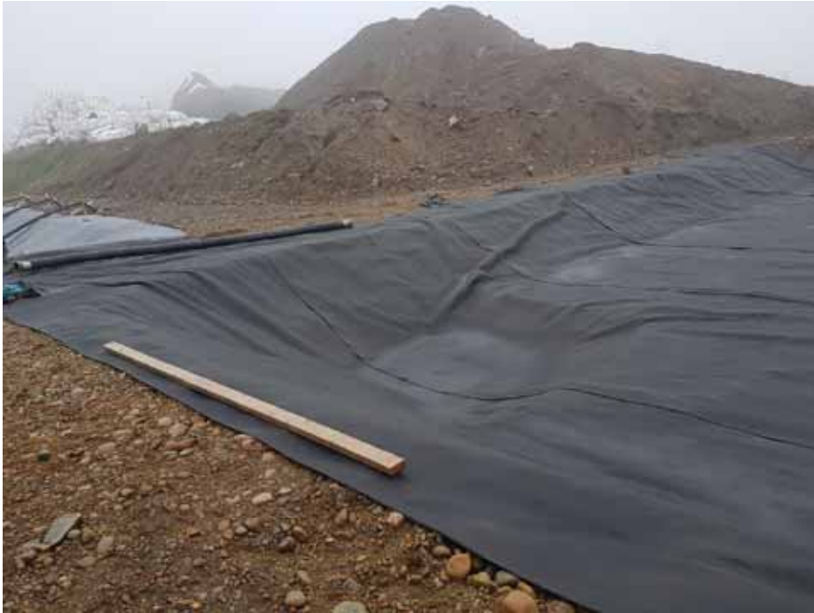
Photo 9 Treated Effluent Holding Pond Geotextile
