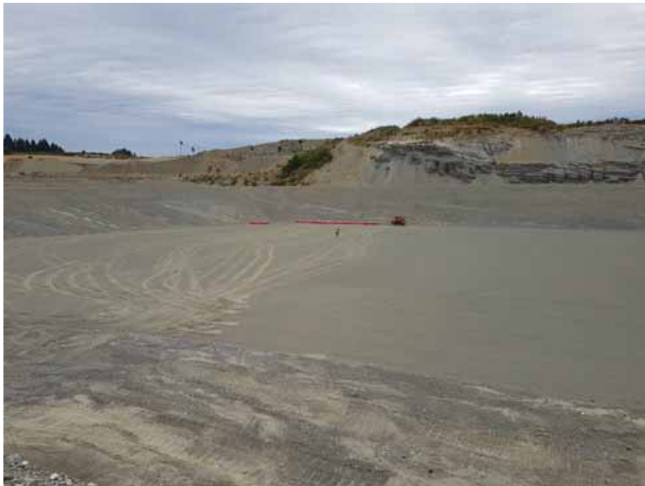
Photo 6 Sub-base Before GCL Installation
