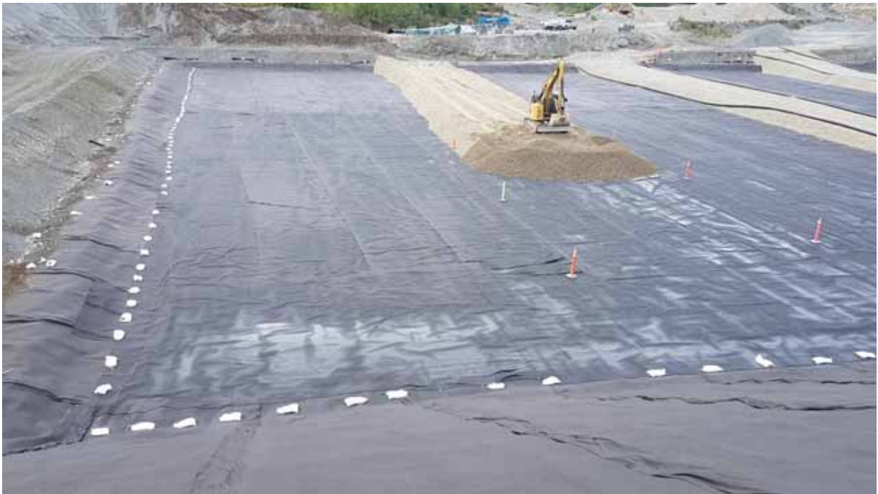
Photo 24 Initial Placement of Drainage Layer in 900 mm Lifts
