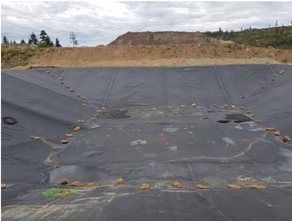
Photo 8 Leachate Treatment Pond Geomembrane Installation Complete
