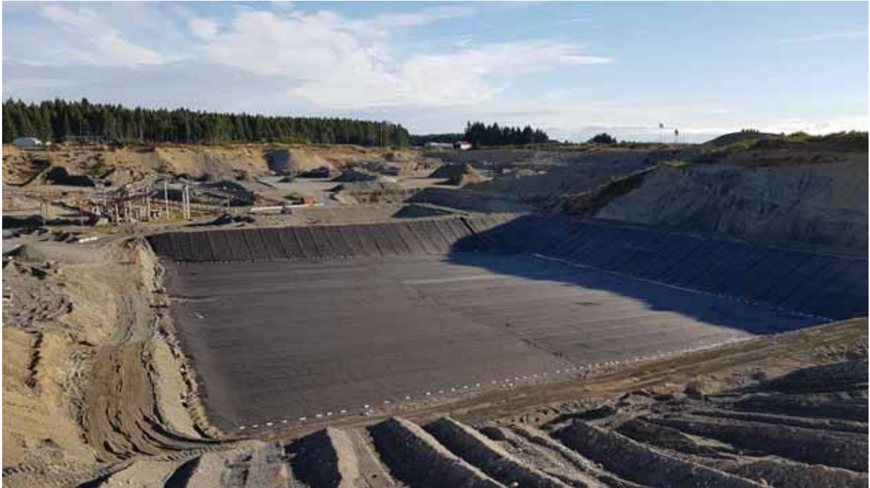
Photo 23 Complete Installation of Geosynthetics
