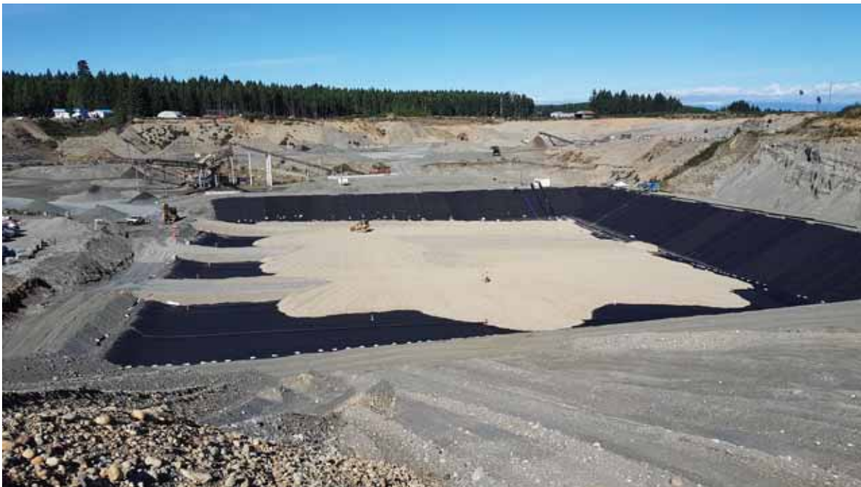
Photo 27 Spreading 300 mm of Drainrock
