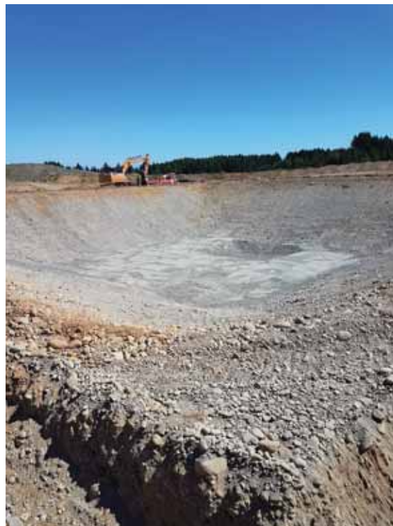
Photo 2 Leachate Treatment Pond Excavation Complete
