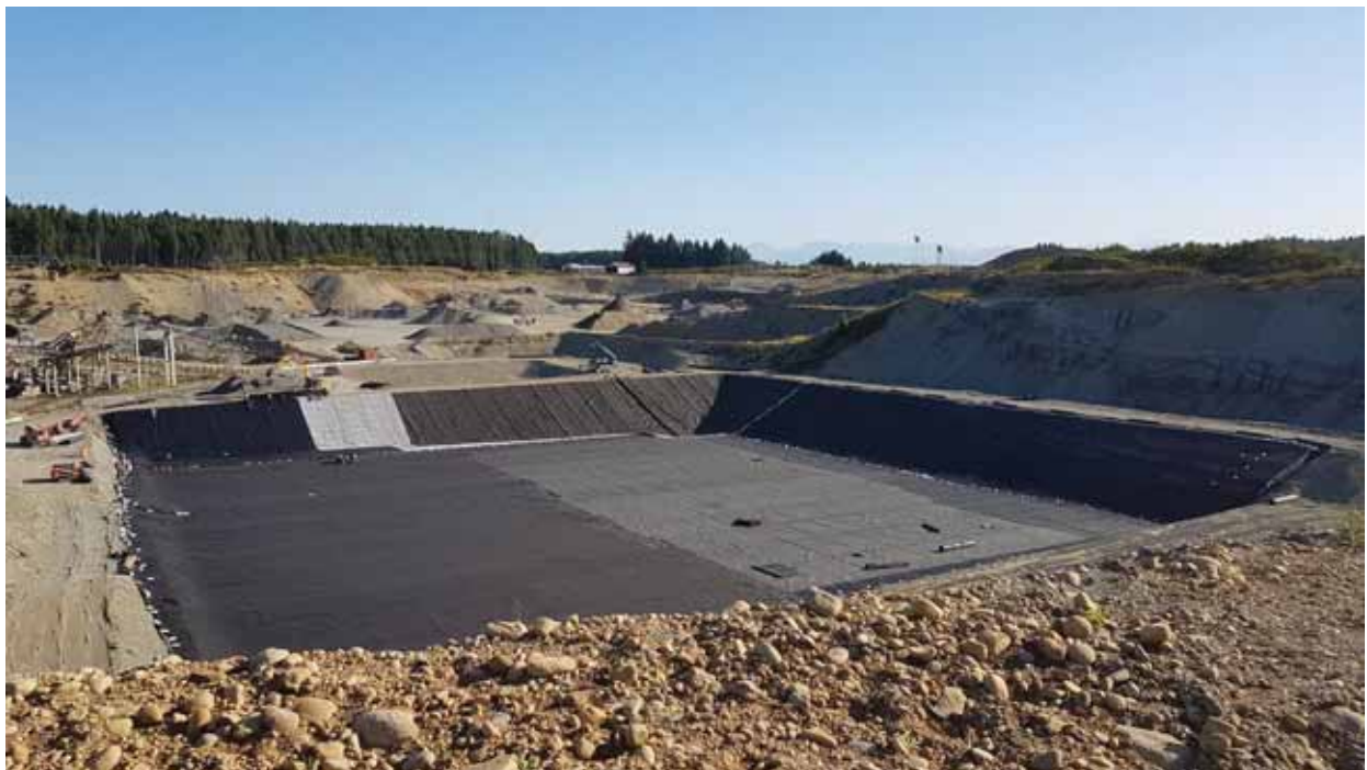
Photo 20 Deploying Geomembrane on North Berm
