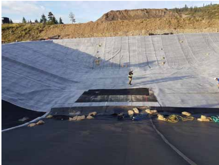
Photo 6 Leachate Treatment Pond GCL Placement
