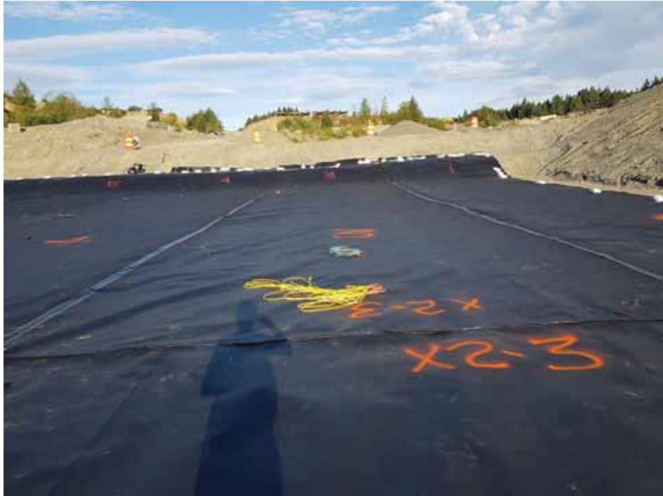
Photo 9 Primary Geomembrane Installation
