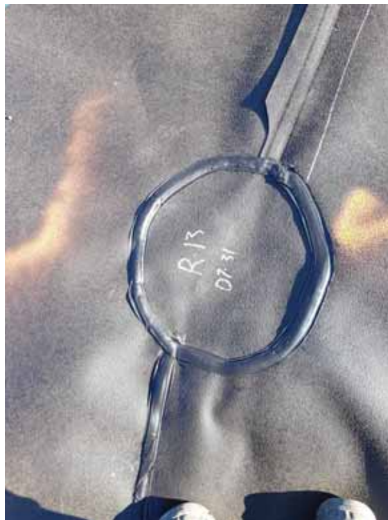
Photo 4 Leachate Treatment Pond Typical Repair
