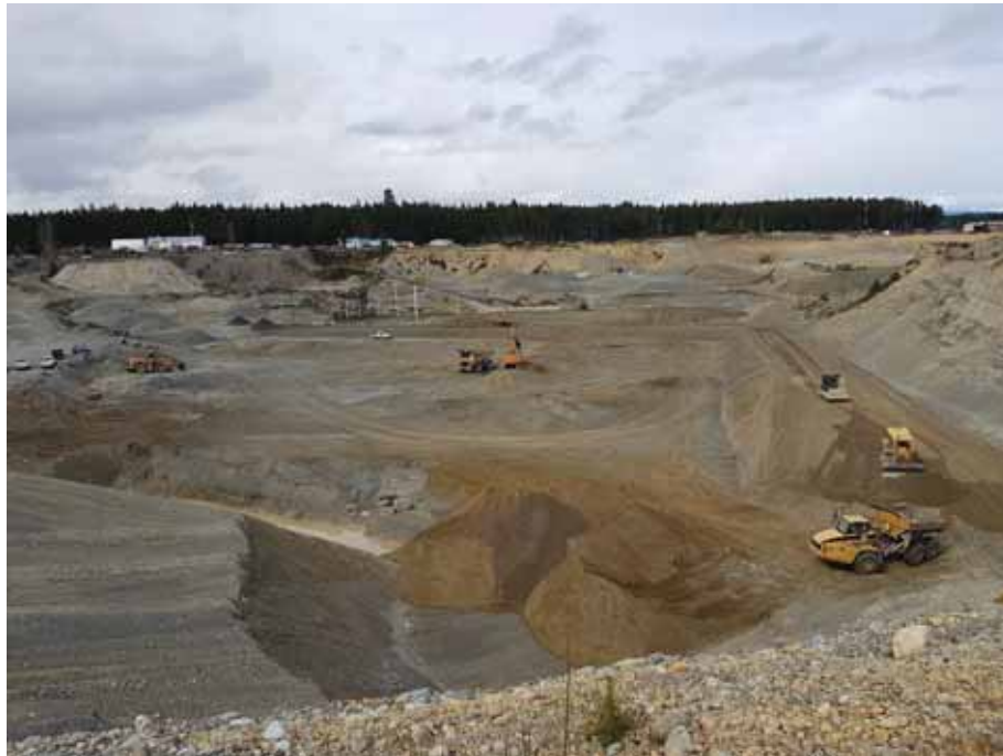
Photo 1 Constructing East and West Berm
