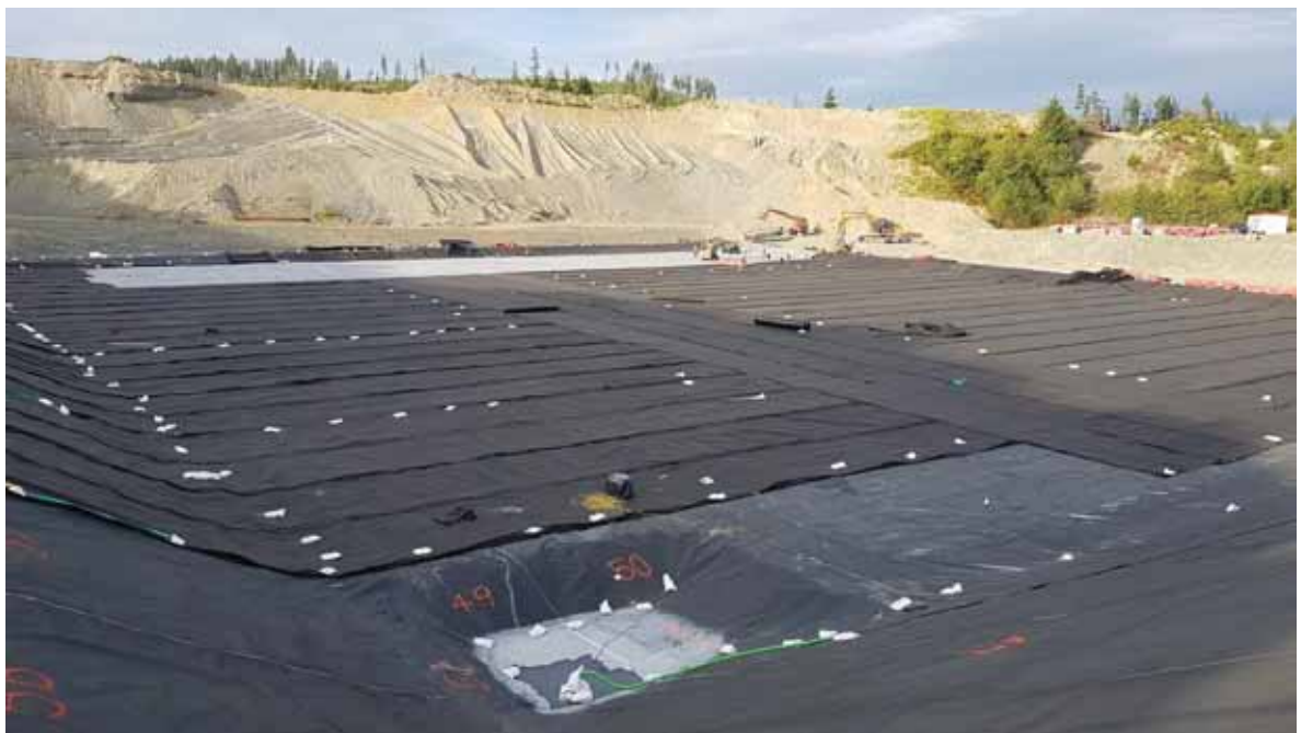
Photo 16 Leachate Sump with Primary Geomembrane
