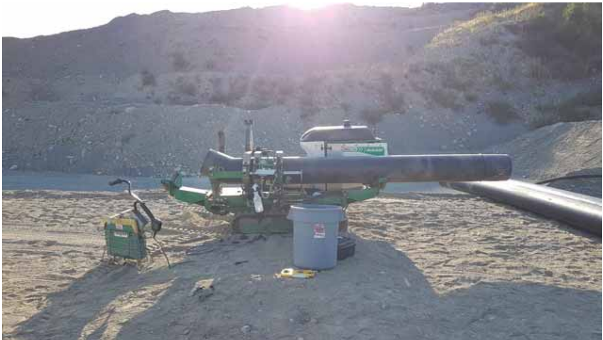
Photo 19 HDPE Pipe Fusion Machine
