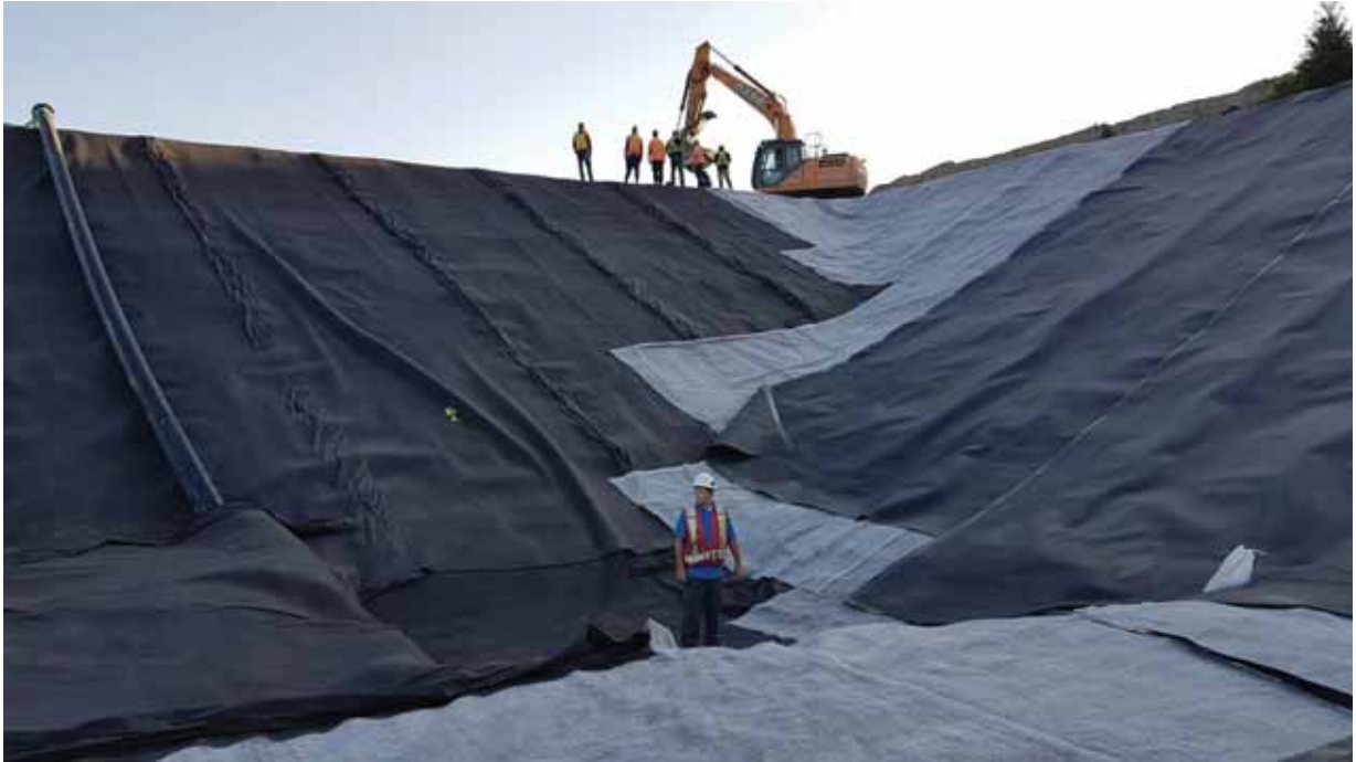
Photo 21 Leachate Sump with Leak Detection Riser
