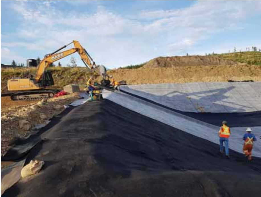
Photo 7 Leachate Treatment Pond Geomembrane Deployment
