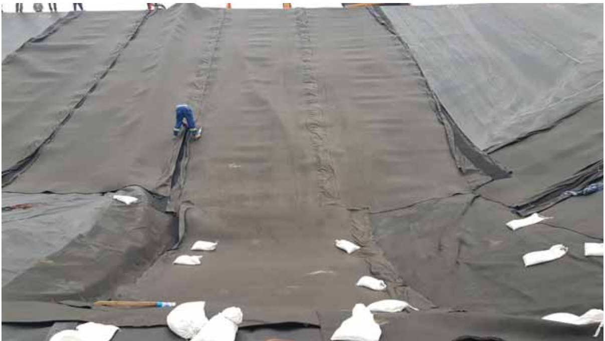
Photo 22 Seaming Geocomposite above Sump
