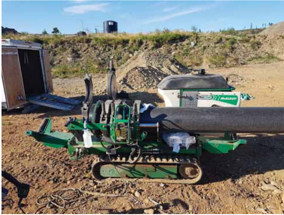
Photo 5 HDPE Fusion Machine
